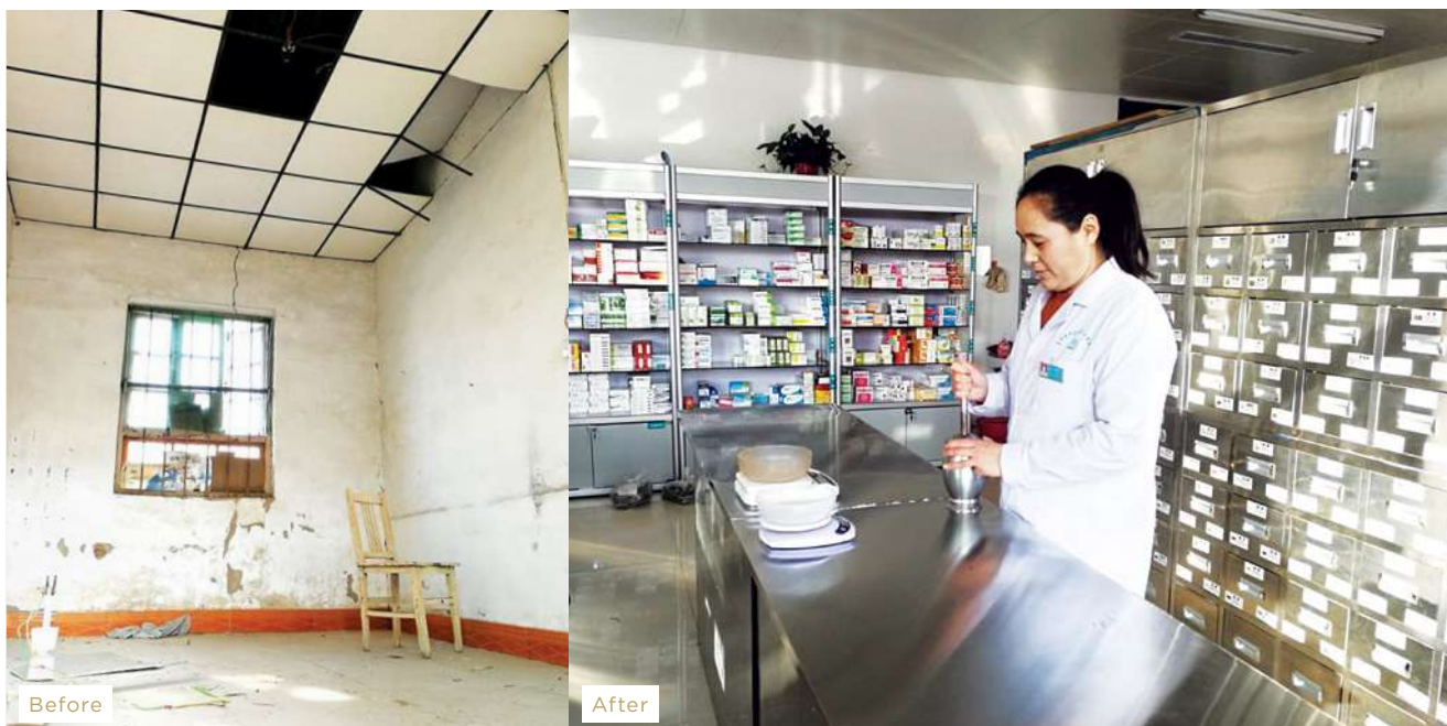
Renovation of Health Service Center
